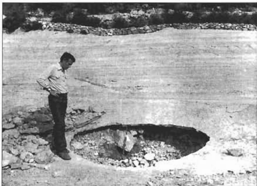
Fig. 5 - Subsidence created in a shotcrete protective layer by strong groundwater uplift.
