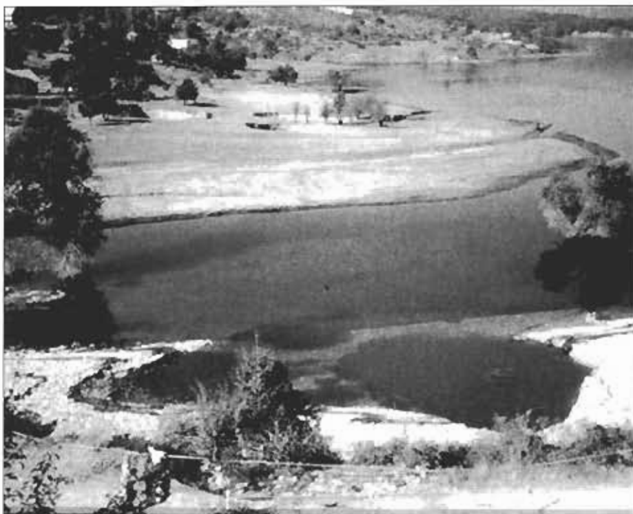
Fig. 9 - Mavrovo Reservoir. Subsidence induced by reservoir operation.
